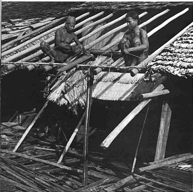
There are no professional carpenters and builders among the Ibans. A man builds and when necessary repairs his own part of the longhouse. If it is a big task he will gladly be helped by his friends. Here two men repair the roof of the ruai where it opens out into the tanju. The roofs are made either of some form of palm leaf thatch or of hardwood shingles. Few nails are used. Everything is tied together with lengths of rattan.
