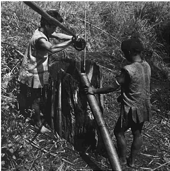
At Ba Kelalan, at the head of the Trusan, there are several salt wells. The salt water is dipped out of the well and carried in lengths of hollow bamboo to a shed where the water is boiled away in large iron pots. Formerly, when access to the coast was difficult and dangerous, such salt wells were an important economic asset and the salt was traded over a wide area. The workers are wearing coats made from bark cloth.
