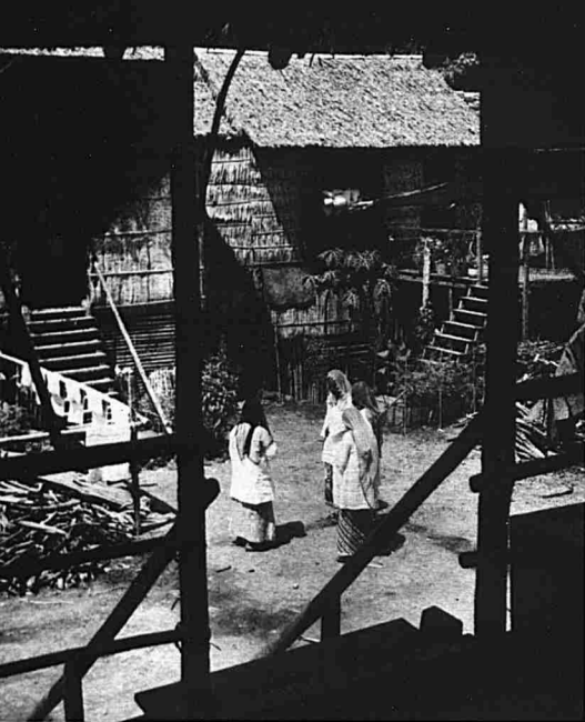
Village scene. The houses crowd one upon another, each one perched on the top of piles, the only possible building system for a people whose houses are generally situated in tidal areas liable to flood. Houses such as these are cheap and simple to make, the walls and roofs being of palm leaf thatch, and they have a useful life of about seven years.
