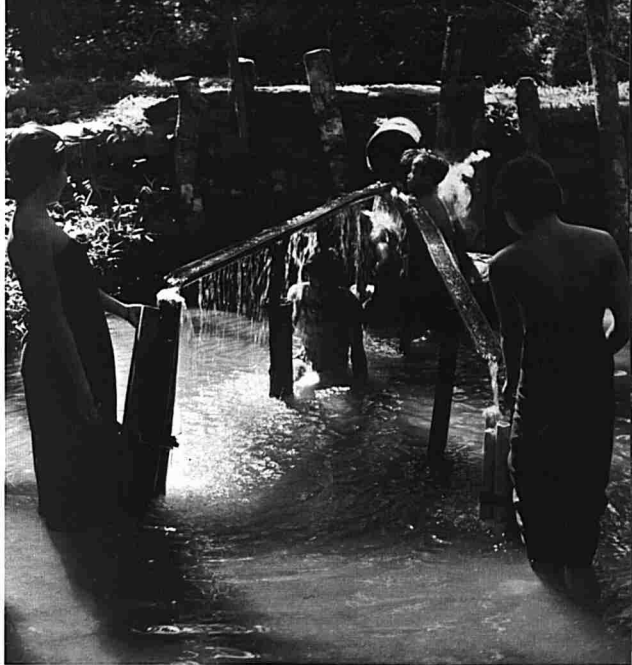
Split lengths of bamboo make useful water pipes and the Land Dayaks are clever at arranging their water supply so that the water receptacles can be filled with as little exertion as possible.
